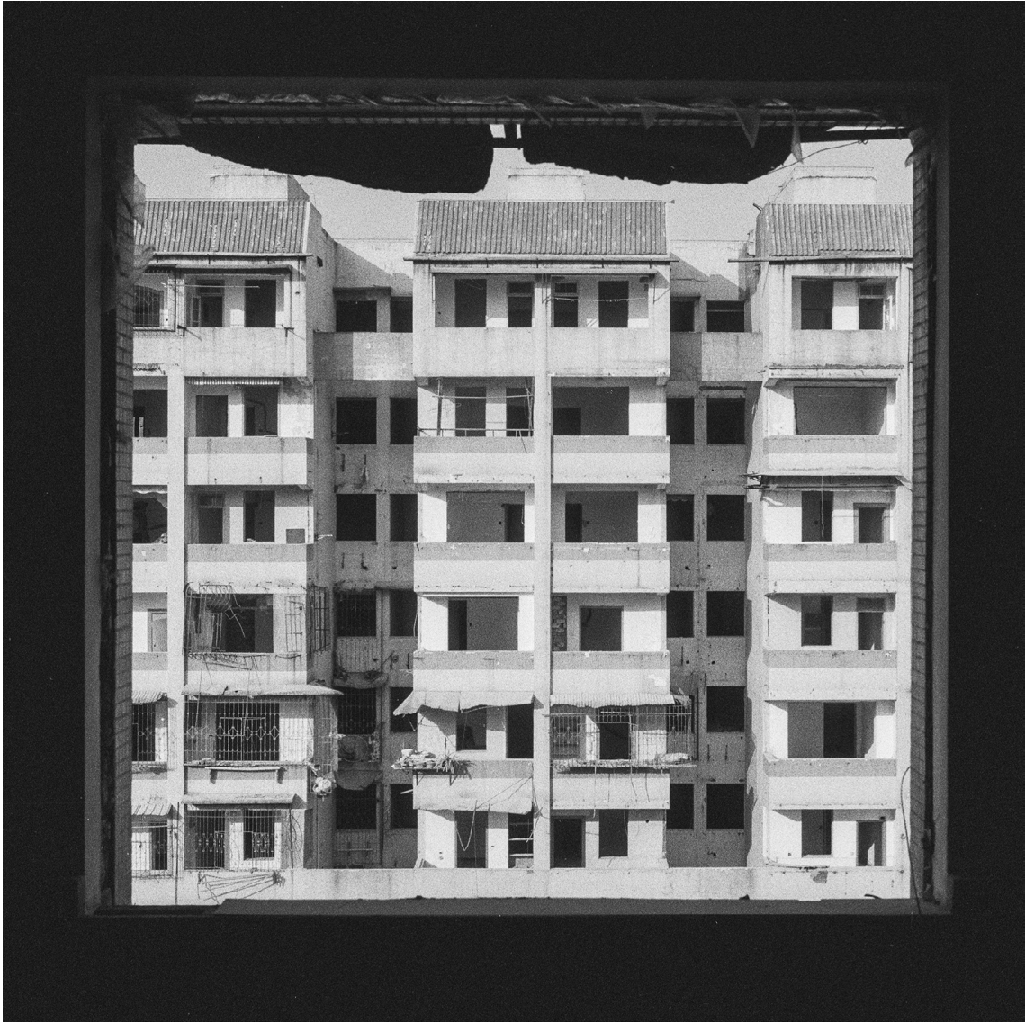
Figure 12. Dust and Scratches : almost all of the ruined building have no glass over the windows; all the windows look like darkened squares from afar.
